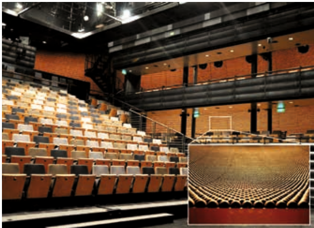
BASF's specialty foam Basotect® is fitted behind approximately 400,000 timber beads which line the curved walls of the unique oval-shaped Genexis Theatre at Fusionopolis, Singapore.
